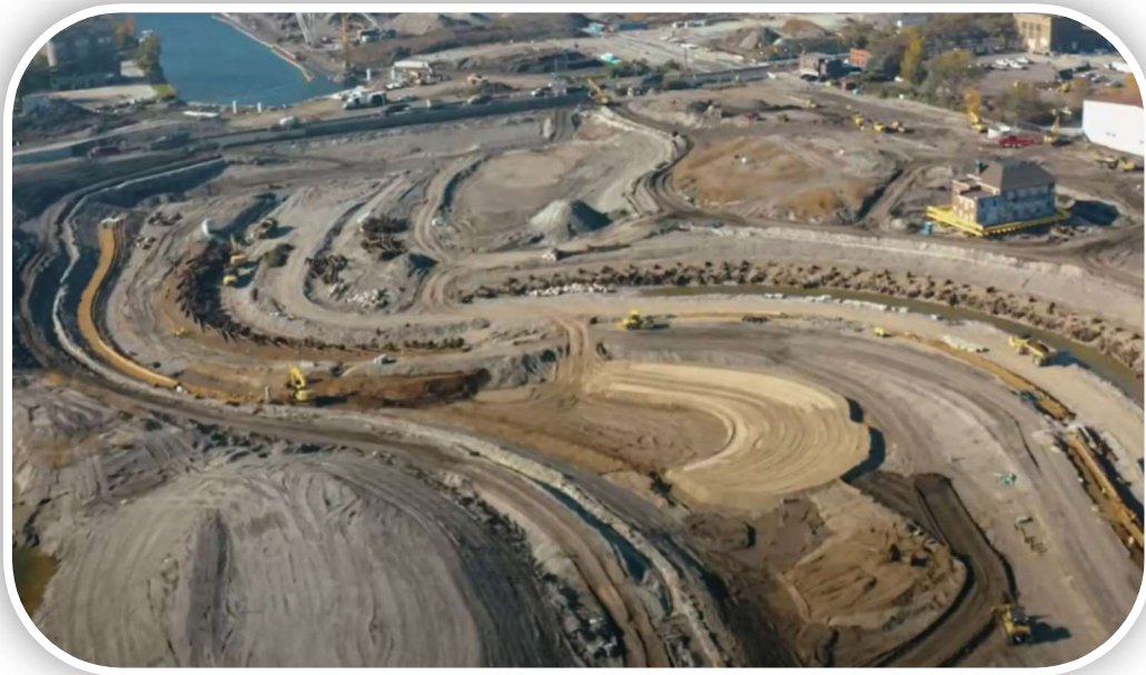
FIGURE 21 CURRENT WORKS OF RIVER REDIRECTION AND FLOOD MITIGATION WORK
