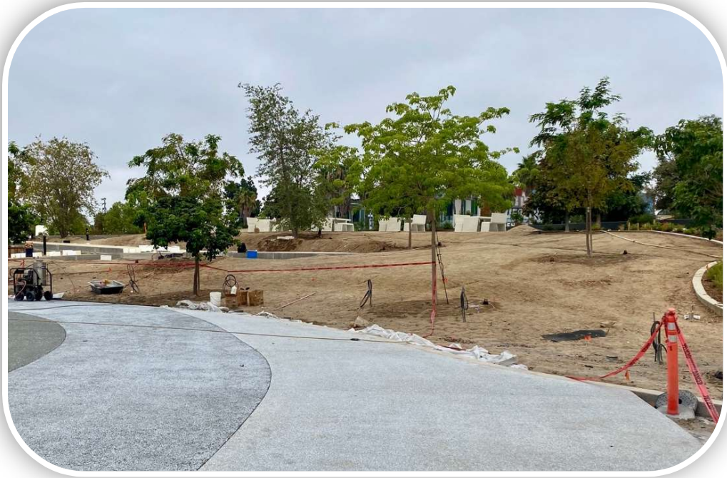
FIGURE 5 LANDSCAPED AREAS ON TOP OF A MULTI-LEVEL CARPARK
