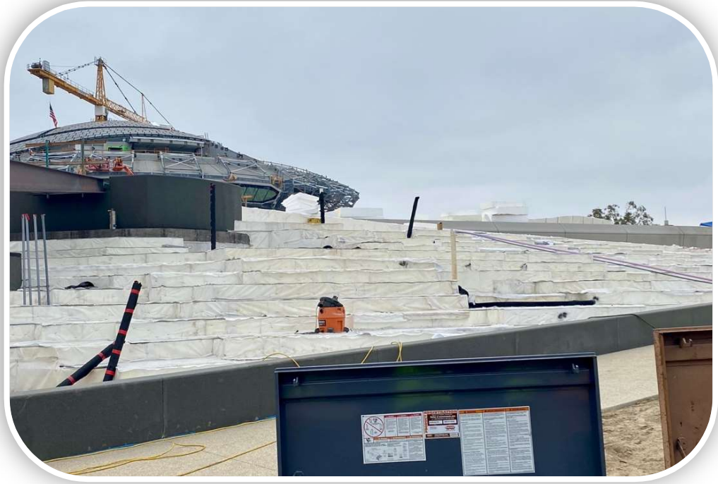
FIGURE 6 GEOFOAM FORMS A LIGHT SUBBASE FOR LANDSCAPE AREAS AND
