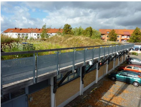
Figure 13 - Demonstration green roof on municipal building in Augustenborg
