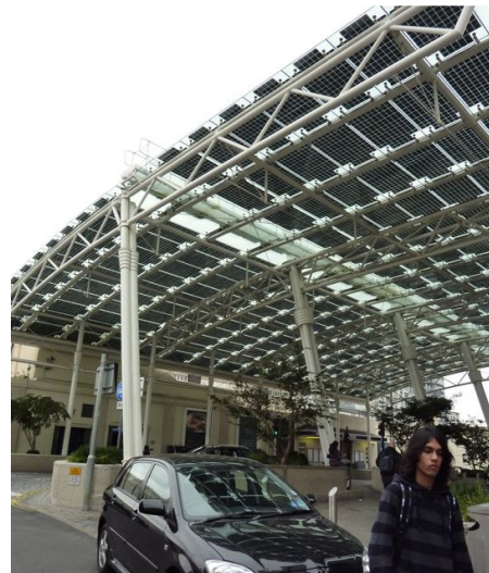
Figure 40 - Albion Square Canopy, Woking
