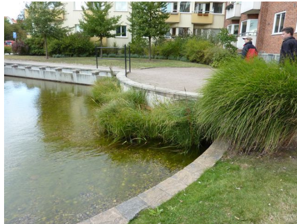
Figure 16 - Open drains feed ponds that help to cleanse storm water and also act as a landscape feature
