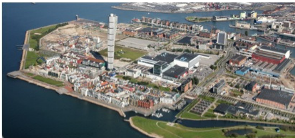
Figure 8 - Western Harbour in 2009, with the Bo01 area in the foreground
