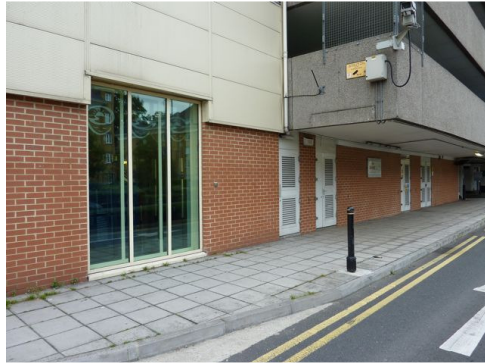
Figure 39 - Woking Town Centre CHP station
