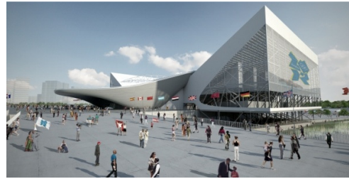
Figure 19 - Image of Aquatic Centre showing temporary stands that will be removed after the Games
