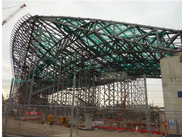
Figure 17 - Construction of the Aquatic Centre's steel frame
