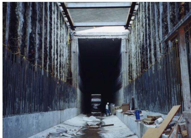
Figure 4-Inside view of wastewater storage/transport pipe
