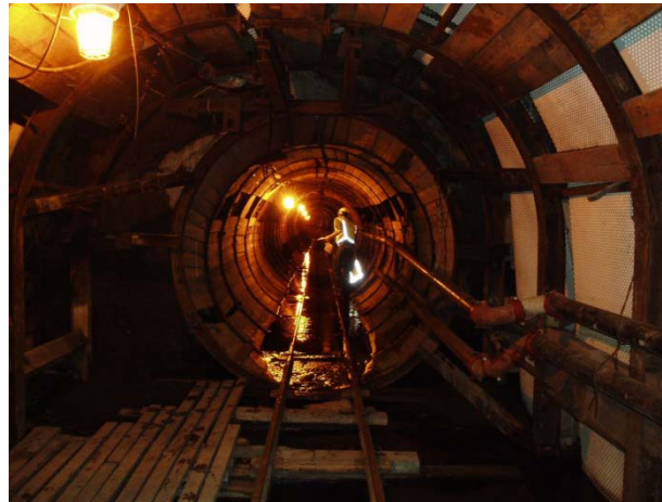
Figure 3-Repairing a defect inside a sewer pipe
