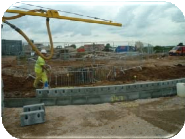
Pre-cast Kerb Construction
