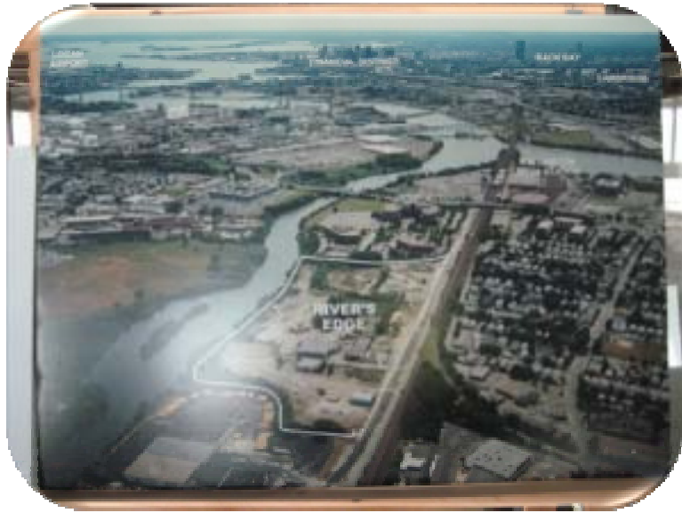
Site of Rivers Edge Commercial Development
