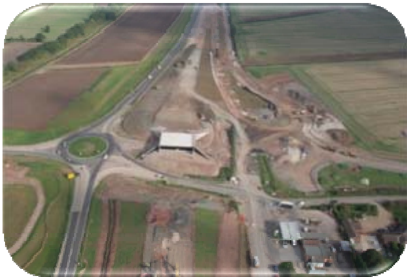
Aerial View of A46 Construction
