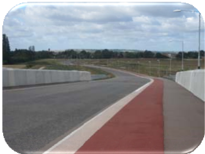
Addingbrooks Access Road
