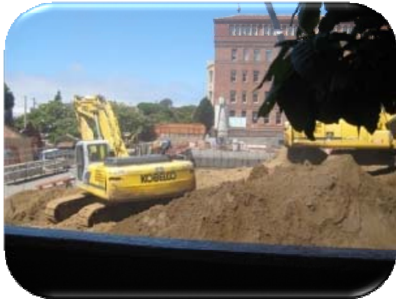
San Francisco General Hospital Construction
