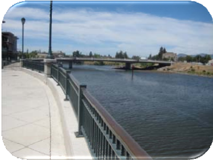
Napa River Bridge and River Frontage Upgrade
