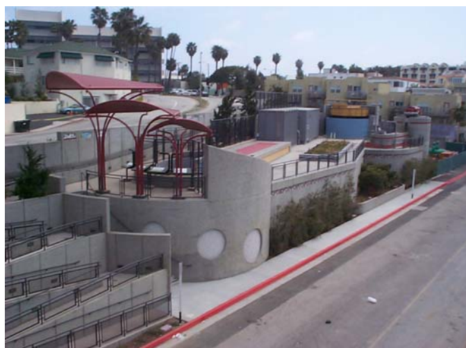
The Santa Monica Urban Runoff Recycling Facility (SMURRF)
