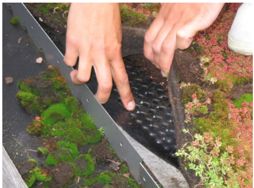
Extensive green roof showing mat and membrane
