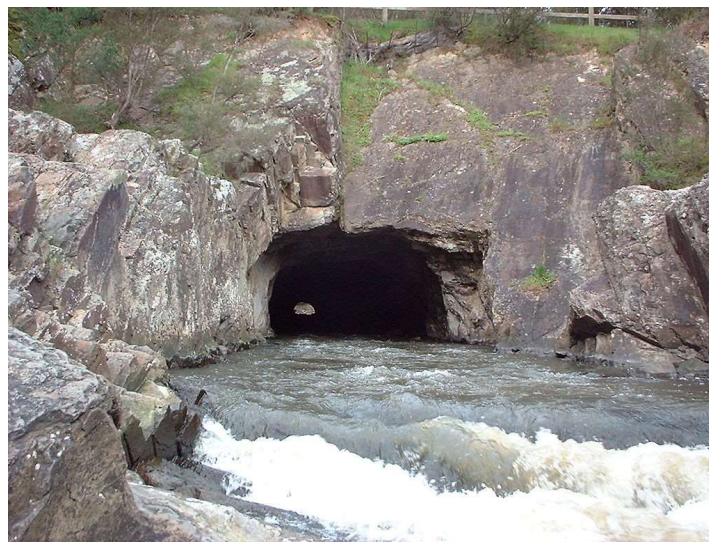
Figure 36 – The historic Pound Bend Tunnel, Warrandyte. The tunnel was constructed in 1870 to divert the Yarra River, so that gold could be mined on the river bed.
