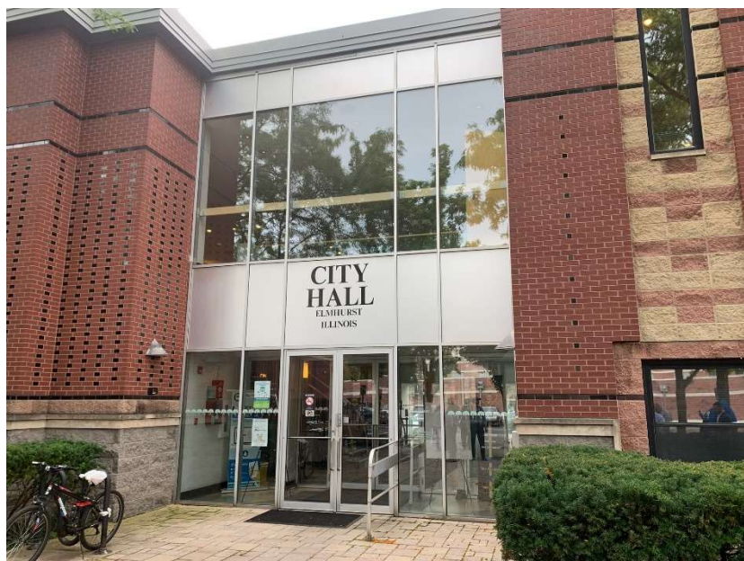
Figure 30 – The City of Elmhurst City Hall
