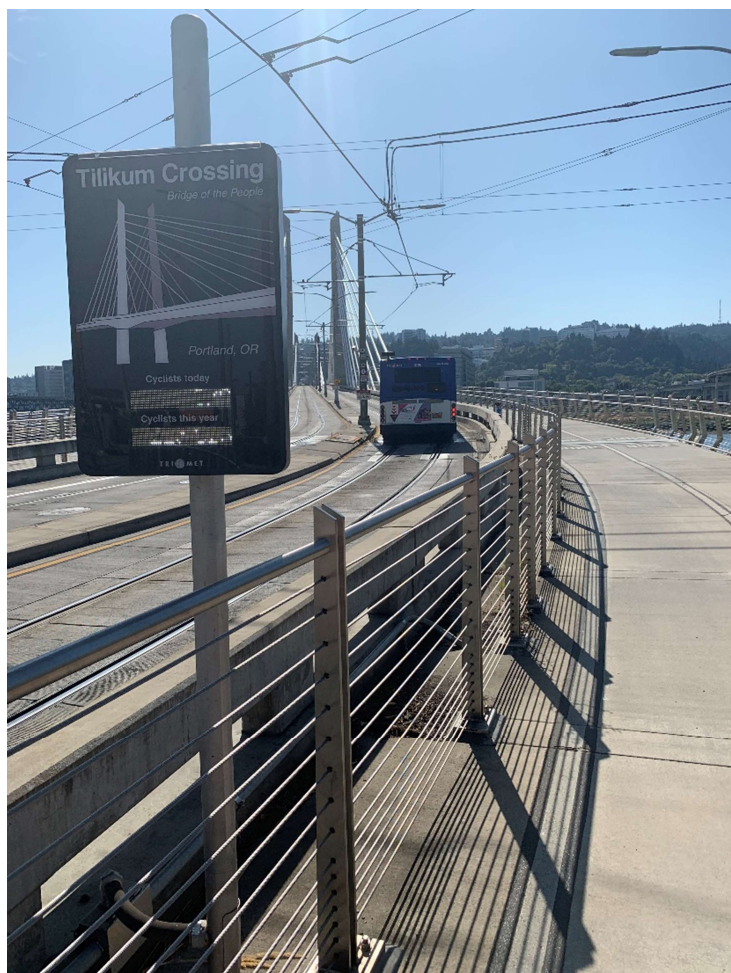
Figure 24 – Tilikum Crossing, Portland, OR
