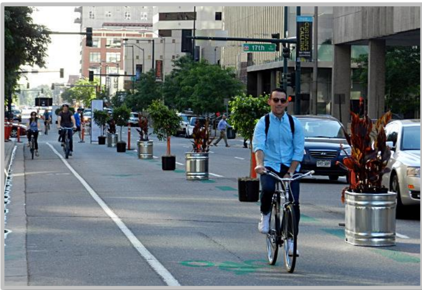
Figure 3: Separate Cycling Lane divided with temporary materials and paint markings
