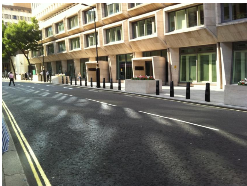
BOLLARDS IN CENTRAL LONDON – BUILT FOR SECURITY BUT AESTHETICALLY PLEASING
