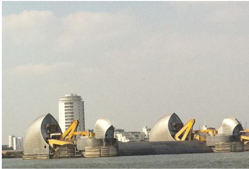
LONDON FLOOD BARRIERS - FUNCTIONAL AND ARCHITECTURALLY AESTHETIC
