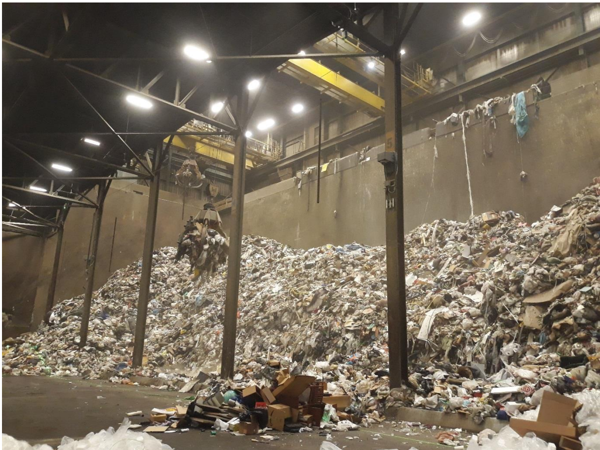
Municipal Solid Waste handling inside the Hennepin Energy Recovery Centre
