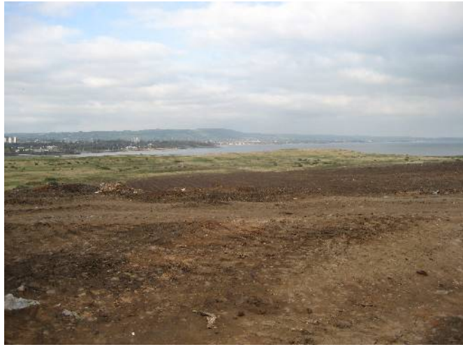
Capping works, Giants Park
