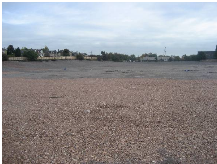
Rehabilitation works, Kenmuir site
