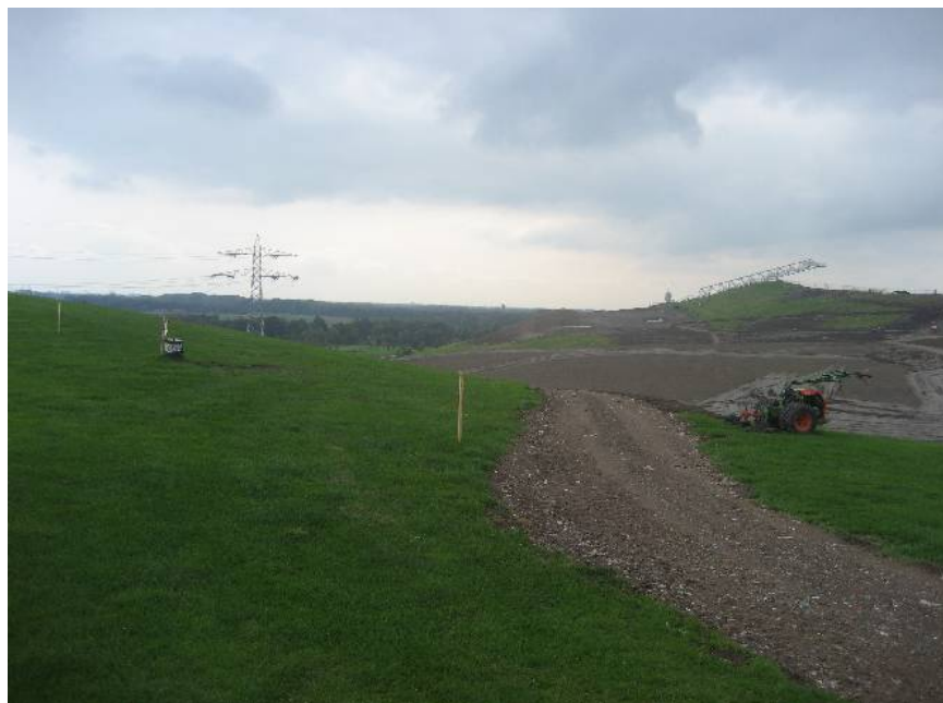
Capping Works – Gulbergen landfill
