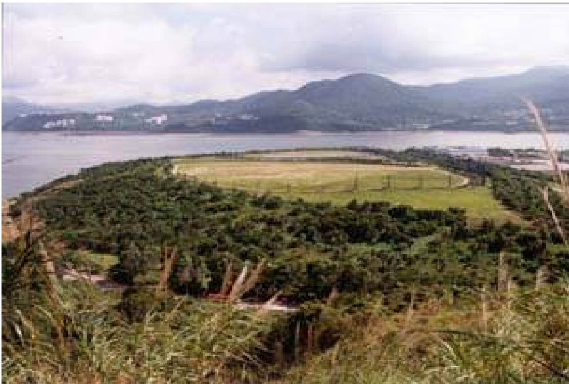
Shuen Wan Landfill (Source: Hong Kong EDP website)
