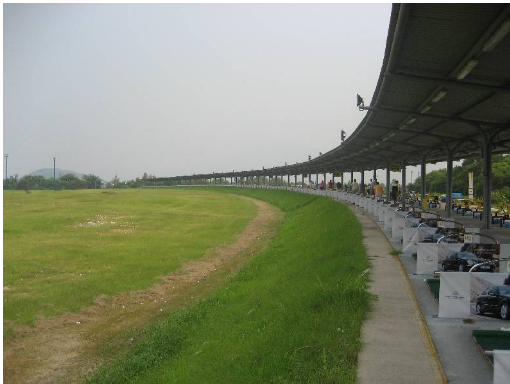
Driving Range Suen Wan Landfill
