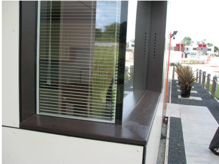
Oxley Wood, Milton Kenes, United Kingdom, September 2008 (Deep wall construction with compressed timber panels on exterior)
