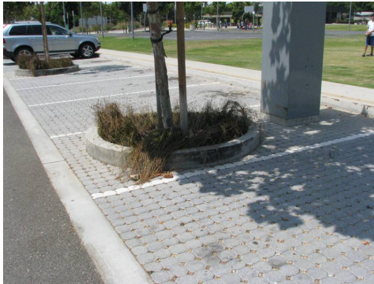
Permeable pavement, Airport Park, Santa Monica, United States of America, August 2008
