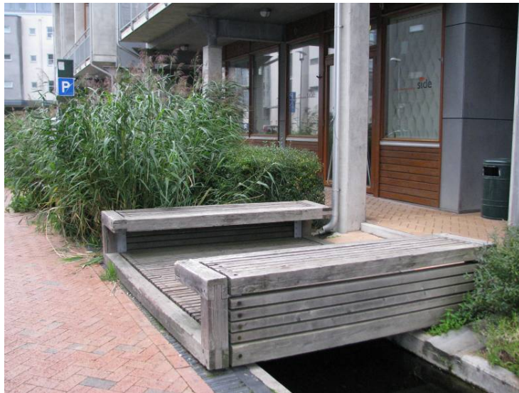
Open channel urban drainage, Malmo, Sweden, August 2008
