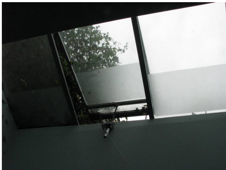
Sutton, London, United Kingdom, September 2008 (Opening ceiling windows)
