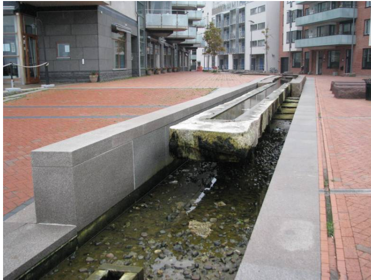
Open channel urban drainage, Malmö, Sweden, August 2008
