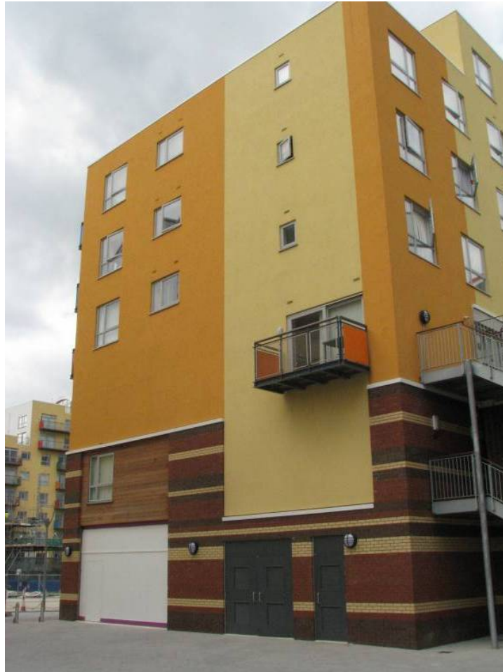
Greenwich Millenium Village, London, United Kingdom, September 2008 (Housing apartment with biomass boiler in bottom corner)
