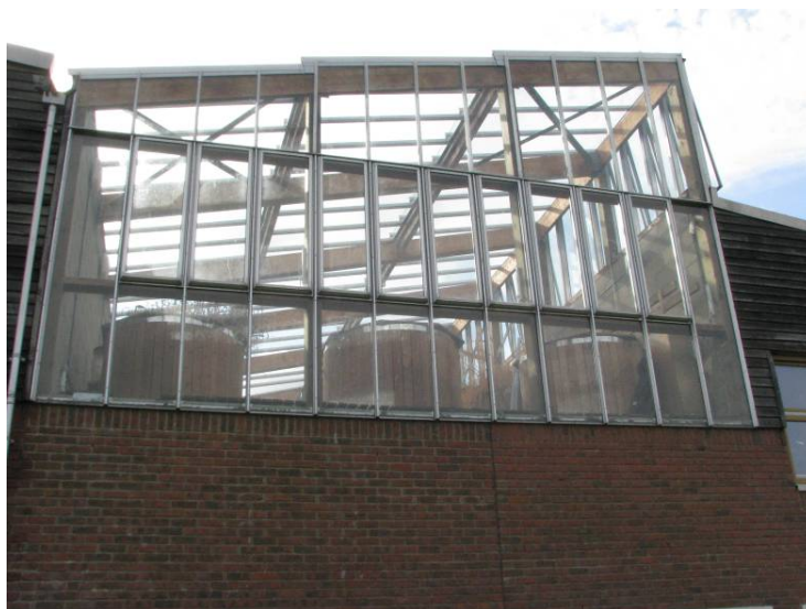
Beddington, Sutton, London, United Kingdom, September 2008 (Wastewater treatment system)
