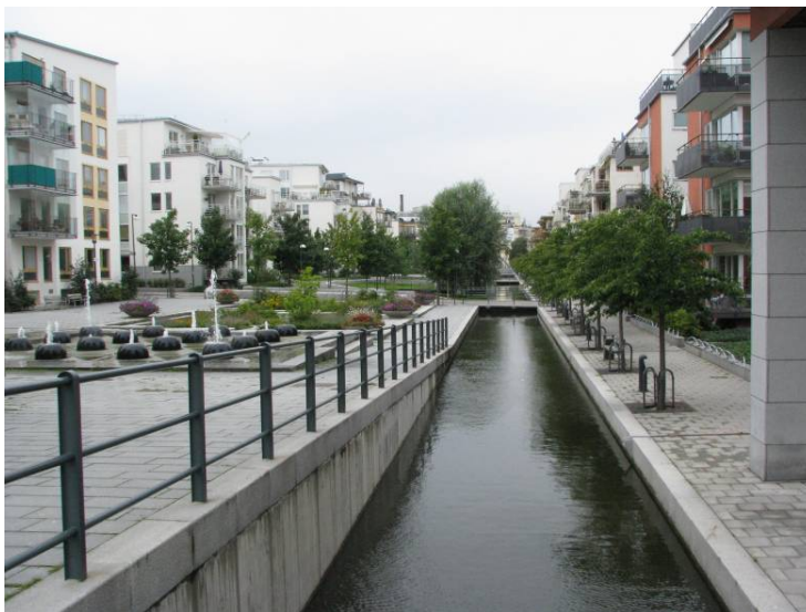
Open channel urban drainage, Stockholm, Sweden, August 2008
