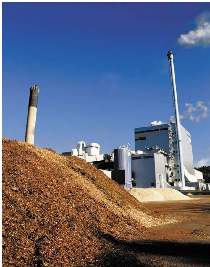
Vaxjo, Sweden, August 2008 (Biomass CHP Plant)
