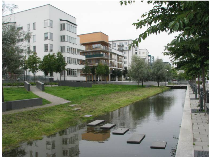
Open channel urban drainage, Stockholm, Sweden, August 2008
