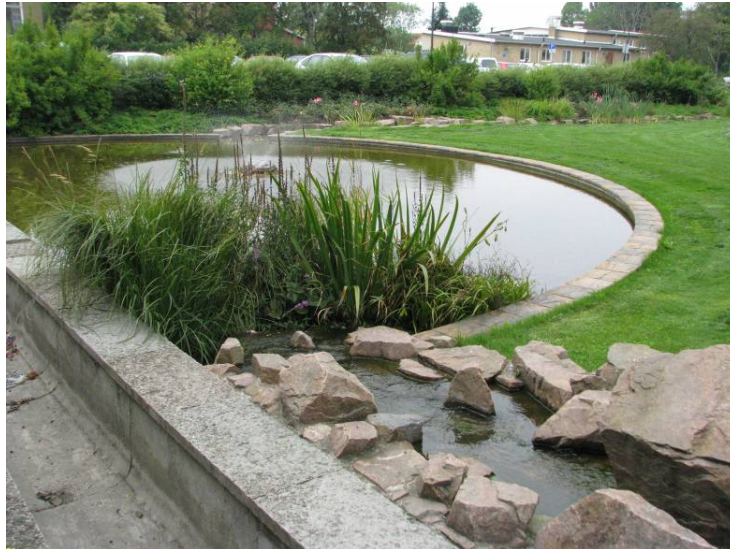
Augustenborgs, Sweden, August 2008 (Surface drainage system)
