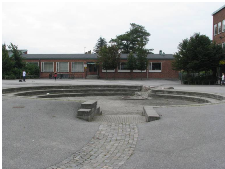
Augustenborgs, Sweden, August 2008 (Surface drainage system)
