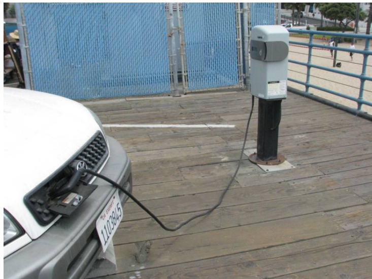
Electric car recharging station, City of Santa Monica Fleet Car, United States of America, August 2008
