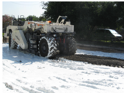
Rehabilitation of road using 30% lime stabilisation
