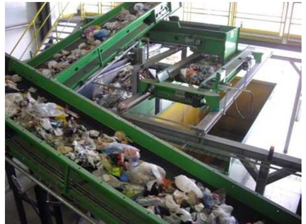
Photo 10 - MBT Plant & Machinery in operation
