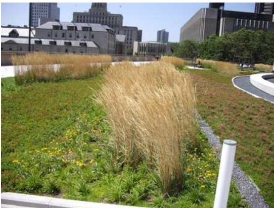
Photo 3 - Green Roof (Toronto City Council)
