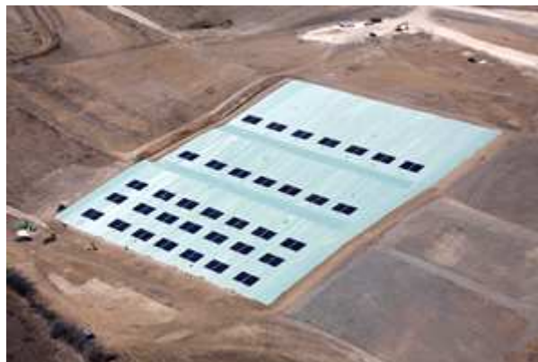
Photo 13- Geo-membrane solar cap for landfill, US
