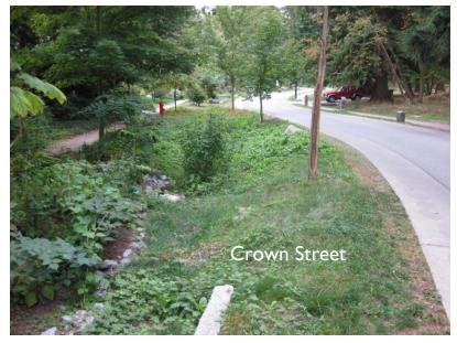
retention swales and concrete edge strips; allowing stormwater to run directly off the pavement, into the swales. The swales then treat the water with natural filtration though vegetation and permeation into the ground. The integrated system is designed with flow and retention capacity for a one in ten year storm.
