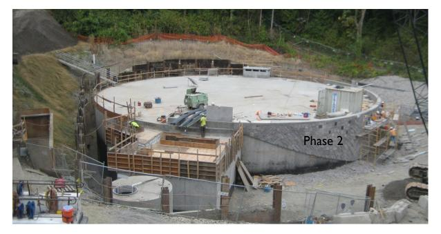
There are no stormwater inlets into the 6.4 million litre phase one retardation basin. Stormwater entering the watershed (catchment) will only enter the basin when the existing system surcharges and backs up through the drainage system. The basin will store water until the drainage system can cope and the stored water will flow out via the 1200mm outlet pipe. The retardation basin is designed for a 1 in 40 year storm event. The total cost for the project is \$30million.
