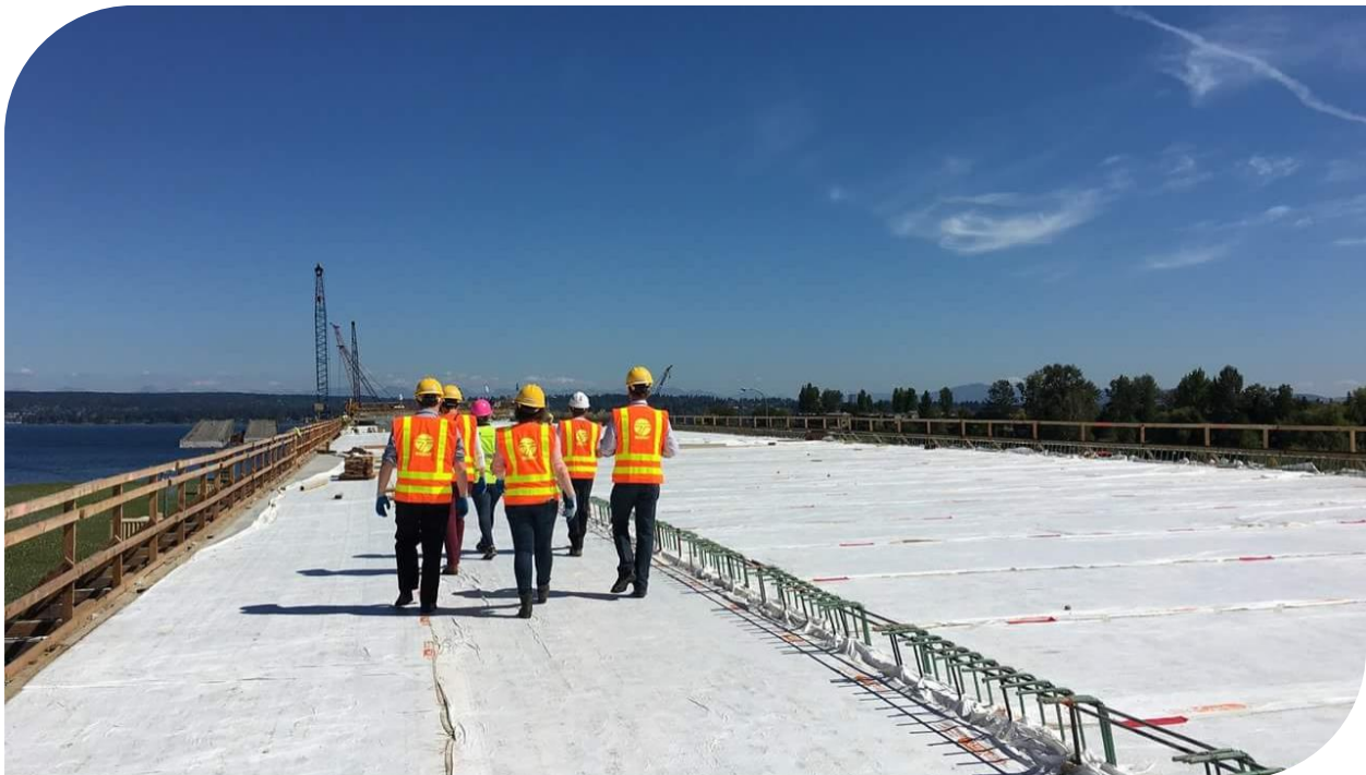
Figure 15 – Onsite at SR 520 in Seattle, Washington, where the new floating bridge is currently under construction.
