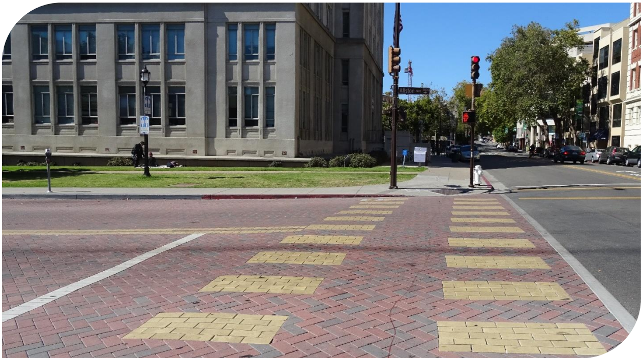
Figure 12 – A trial pavement project in the City of Berkeley, Allston Way, which allows stormwater runoff to infiltrate through the road and into the underground water table.
