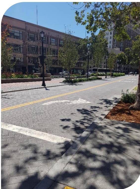
Figure 4 – Telegraph Avenue, in the City of Oakland, is a recent Complete Streets project which was reopened to the public in May 2016.
