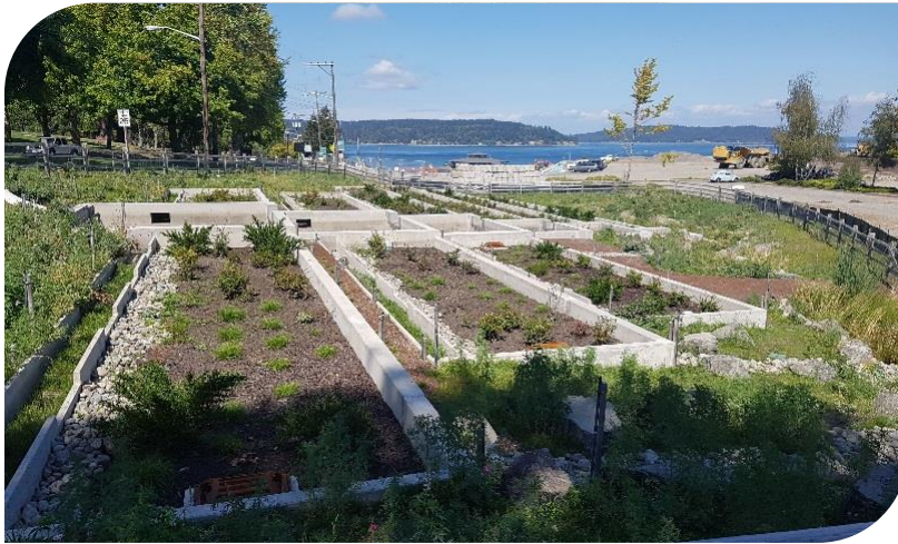
Figure 8 – Point Defiance Regional Stormwater Treatment Facility, City of Tacoma
