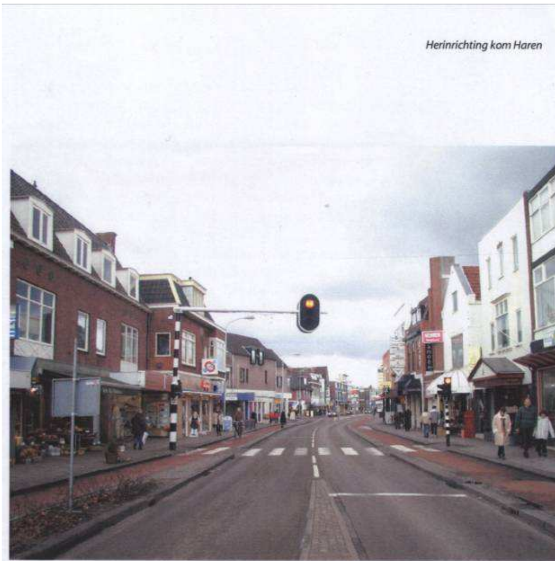
Figure 11 - Rijksstraatweg, Haren before reconstruction. Separate cycle ways, narrow footpaths, two way road with white line.
