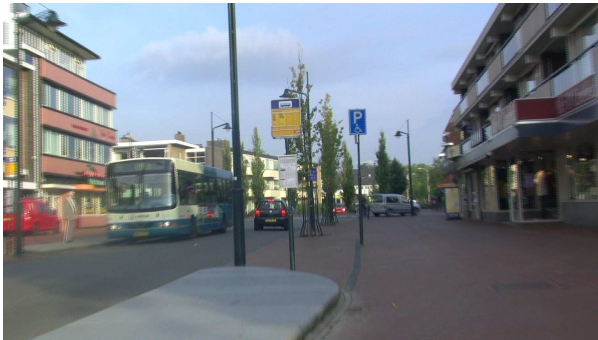
Figure 20 - Raised concrete bus stop
