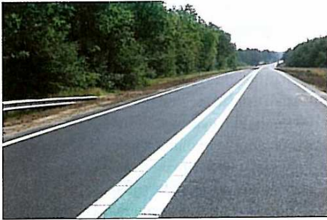
Rural Through Road (Main Road) –Netherlands (Regionale stroomweg type 1 1x2 – refer to Table below)
