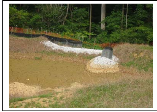
Sedimentation Construction Pond
