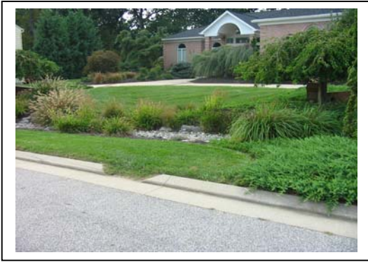
Rain Garden in Local Street
