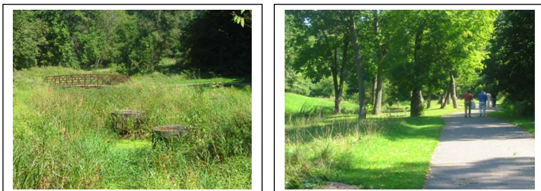
Battle Creek Erosion Control Project – 1.100 year pipe system below creek bed.
