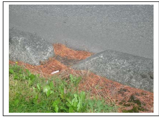
Bio-filtration Swale With Kerb Openings Within Median of Main Road
