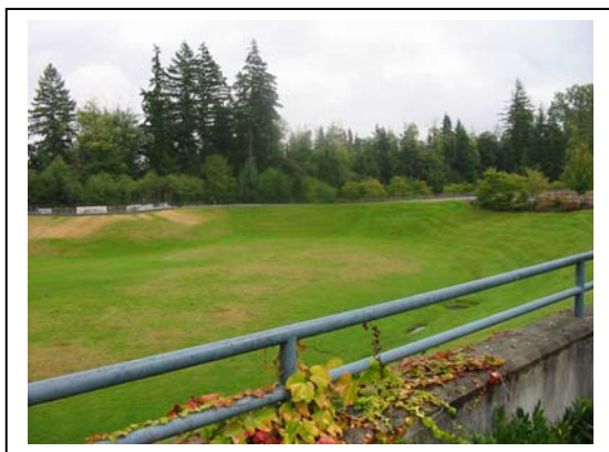
Neighbourhood Detention Facility
