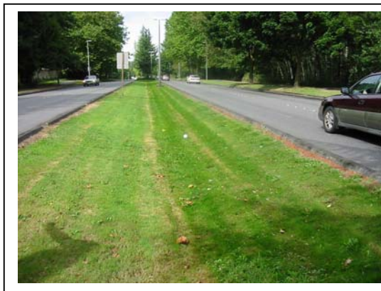
Bio-filtration Swale With Kerb Openings Within Median of Main Road
