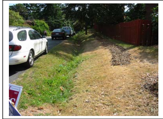
Grassed ditch Pinehurst neighbourhood.
