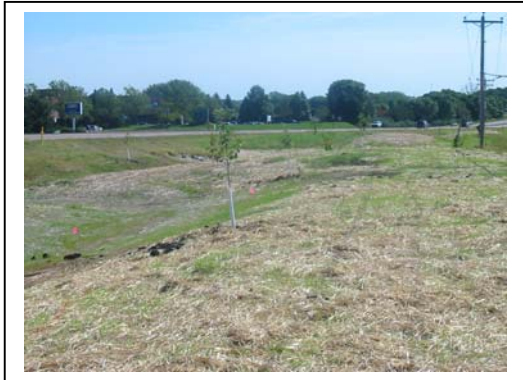
Valley Creek Project – Infiltration / Filtration (Rain Garden) adjacent to Arterial Road.
