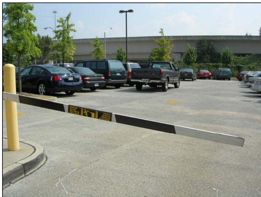
Car park with a porous pavement – City of Atlanta
