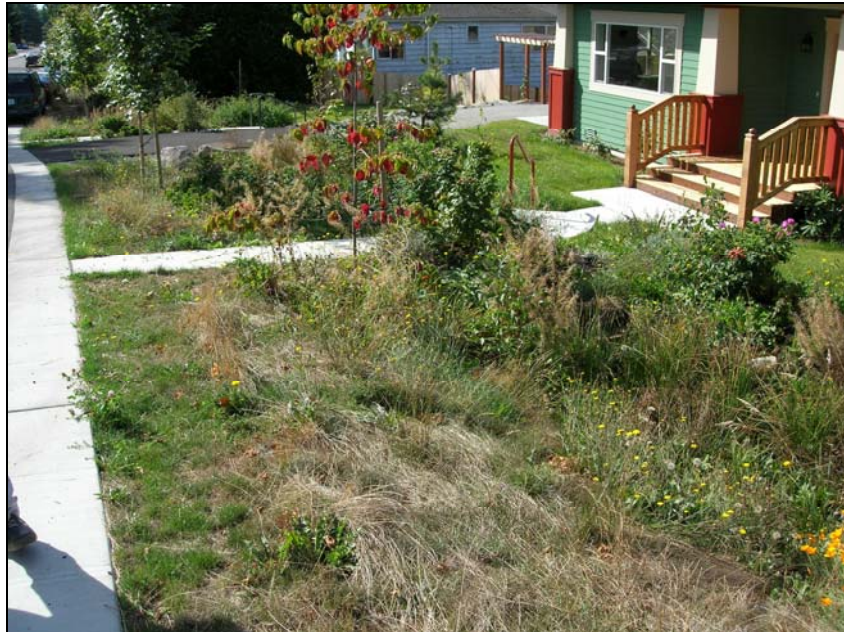
Natural Drainage System Swale – City of Seattle
