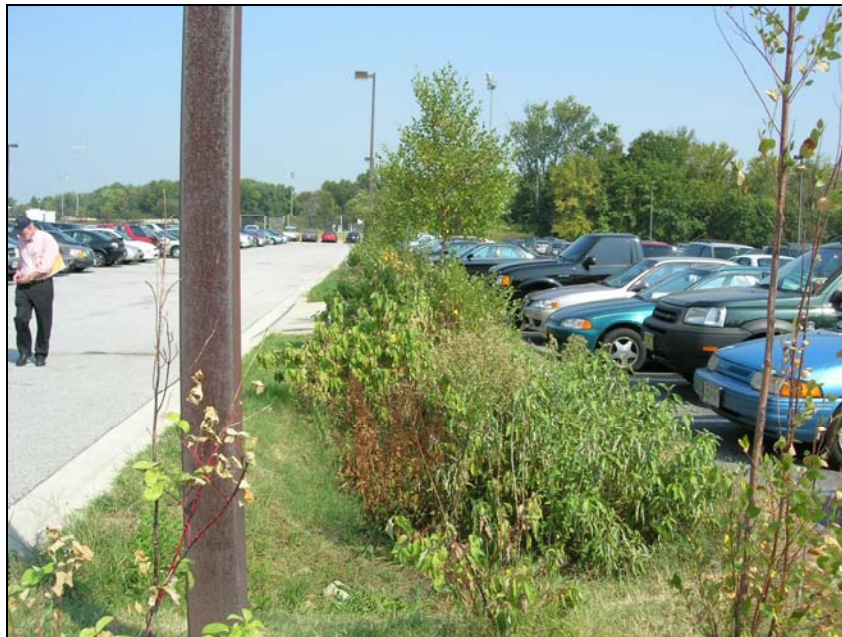
Bio-retention swale in car park at Maryland University - Baltimore
