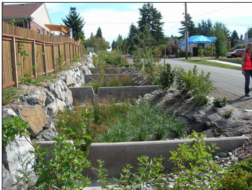
Deep swale posing a potential safety hazard. Natural Drainage System – City of Seattle
