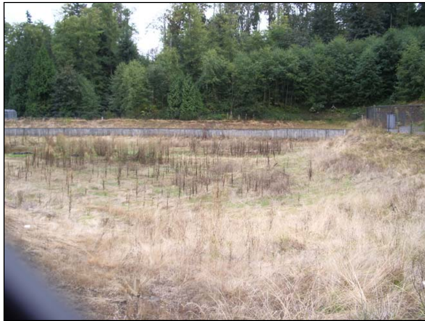
Sand Filter – City of Bellview
