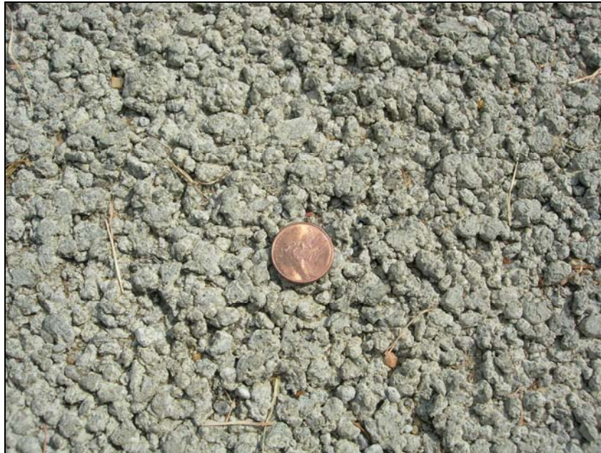
Close up view of porous concrete pavement
