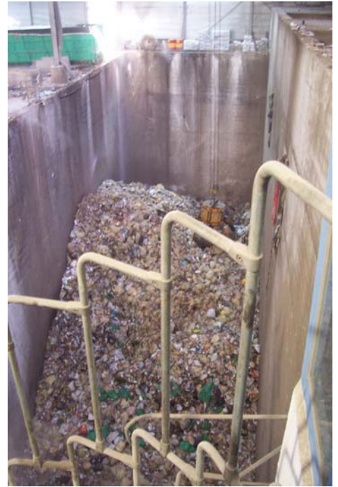
Waste Holding Bays
