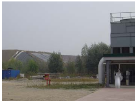
Landfill at Rear of Plant
