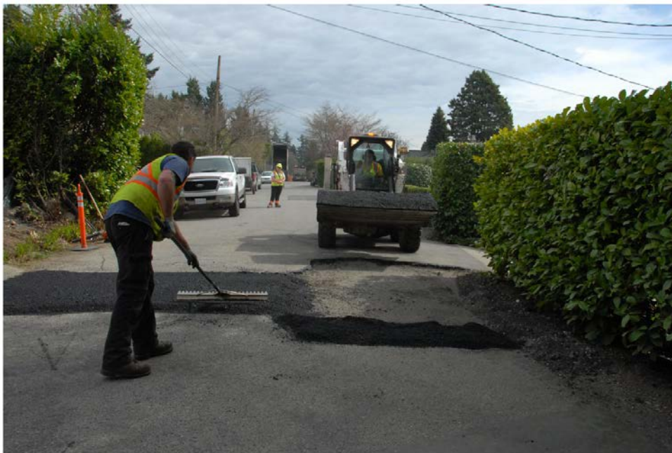
Figure 5 – Road repairs in the District of West Vancouver
