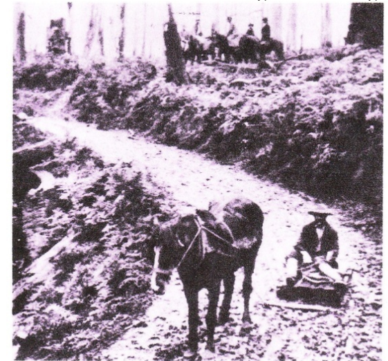
GIPPSLAND settlers contended with "roads" like this. Cedric Tuxen and early CRB engineers faced primitive conditions.
