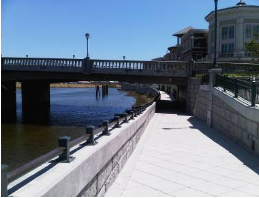
Flood wall turned into a landscape feature used to beautify the city
