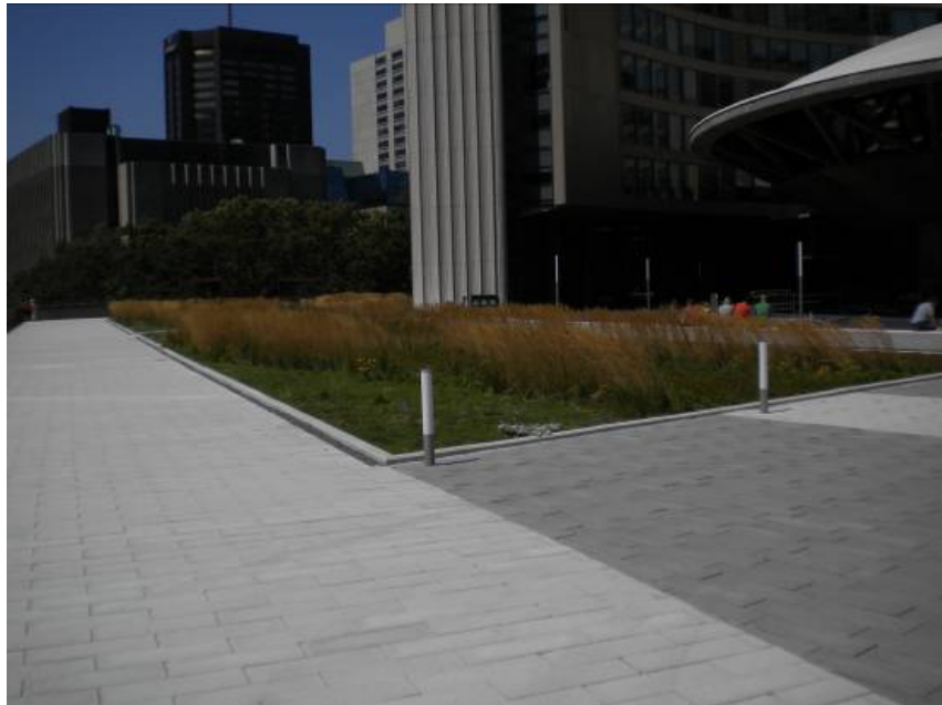
Green Rooftop above the City of Toronto's Council Building
