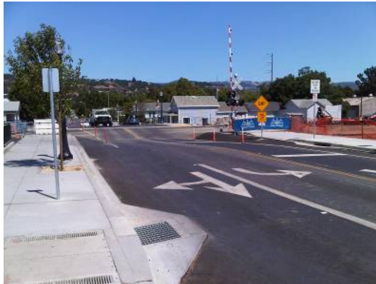
No attempt to restrain or guide the public from entering the construction site
